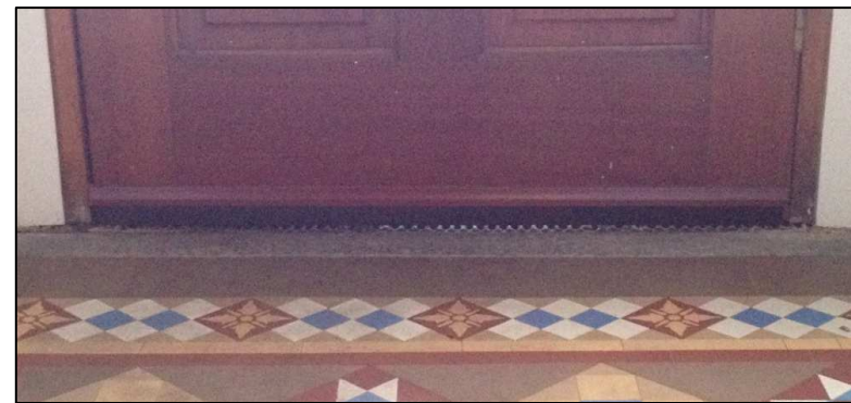
Draught-proofing strips can be easily applied to interior side of external door
